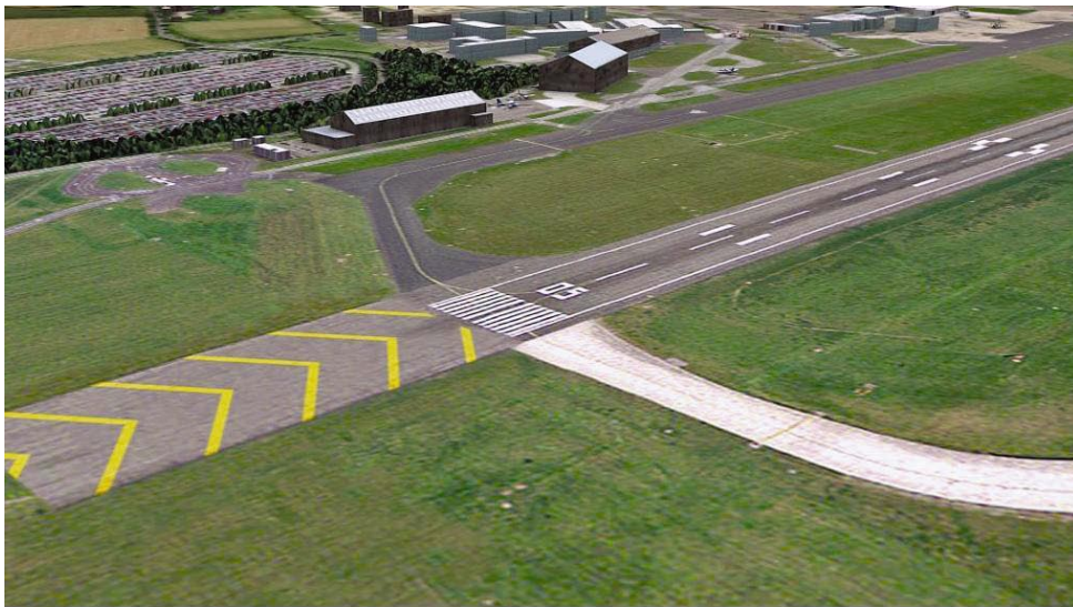
Figure 2.2 Stopways are able to support the aeroplane during an abortive take-off and are marked by large yellow chevrons.
